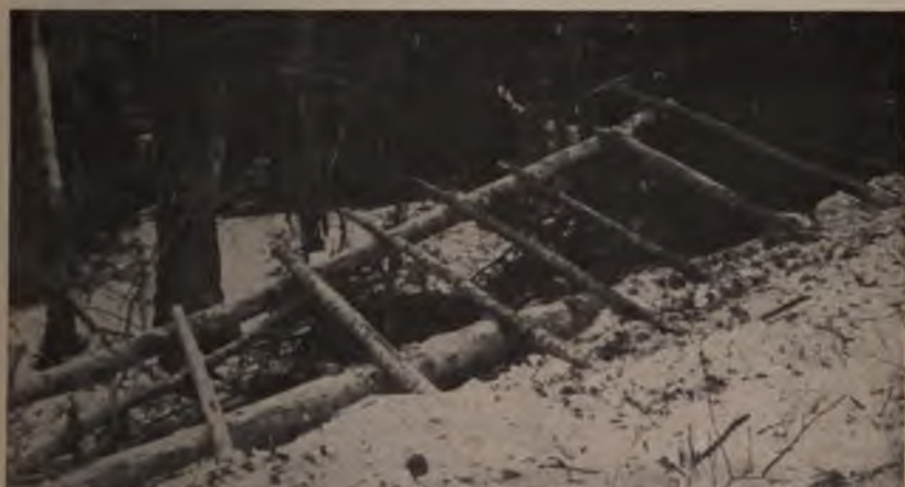
FIG. 38. — A Yarding-sled Road built up on a Curve to prevent the Sleds from leaving the Road. Maine.
